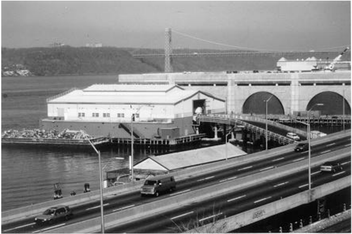
The North River Sewage Treatment Plant.
